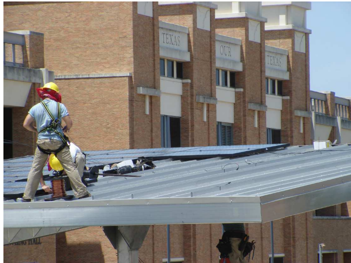
Fig. 01 The University of Texas at Austin first Solar Photo voltaic installation on the main campus, installed as shading devices on the top of Manor Parking Garage (Image Source: Fred C. Beach, Ph.D.)
